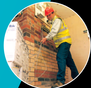
Cabling Media and Infrastructures
